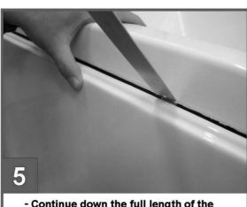
Continue down the full length of the bath using the same method until the panel is suspended by the clip system. (See picture 6)
