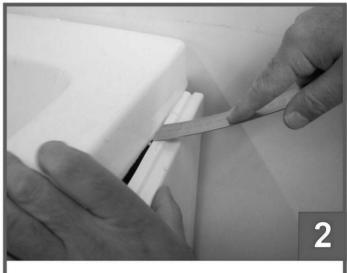
Using a metal ruler or paint scraper push down on the clip while pushing the panel inwards. (See picture 2)
